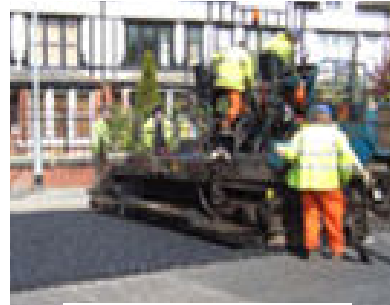
Highway repairs Leeds
